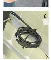
Almost all modern PV modules come with prewired, multicontact (MC) connectors. These connectors simply plug together, allowing fast installation and a low-resistance, weather-tight connection. MC connectors should be firmly pushed together and given about a quarter turn to make sure the seal is tight. Your system design will determine how many modules will be wired in series, and how many series strings your array will have. (See my article on wiring configurations for a PV array in *HP87*.)
